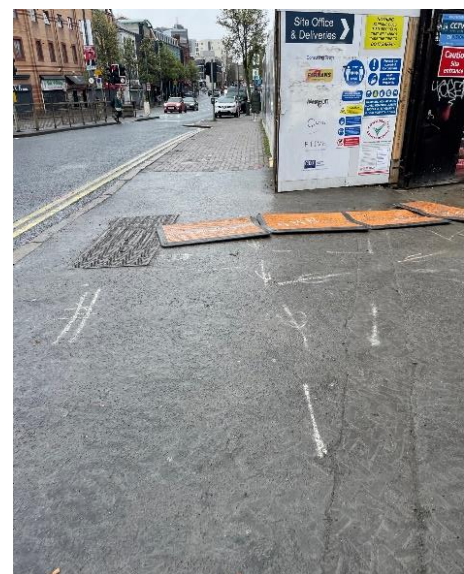
Figure 109: Road works, Shaftesbury Square
