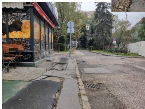
Figure 119: Cracks, uneven paving and standing water, Szeged Hungary
