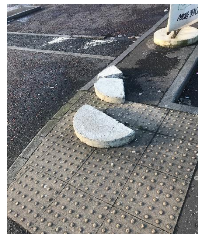
Figure 131: Obstruction on tactile paving, Belfast
