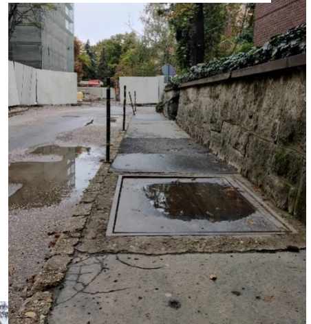
Figure 119: Cracks, uneven paving and standing water, Szeged Hungary
